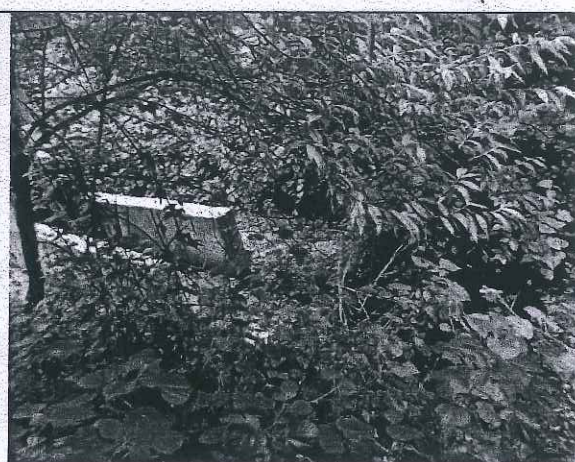
库尾右支线排水斜槽
